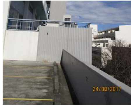
2. Carpark adjacent to parapet
