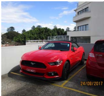
3. Carpark adjacent to parapet wall
