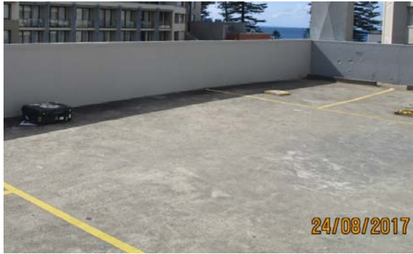
1. Carpark adjacent to parapet wall
