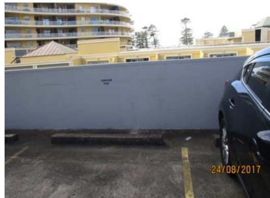
4. Carpark adjacent to parapet wall
