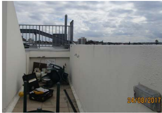
8. North balcony adjacent to solar panel
