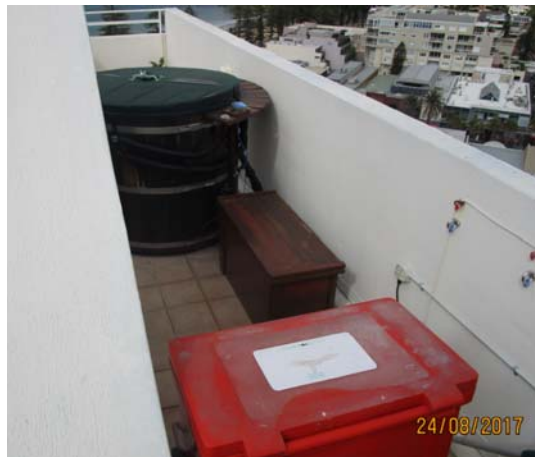
10. South balcony adjacent to water tank
