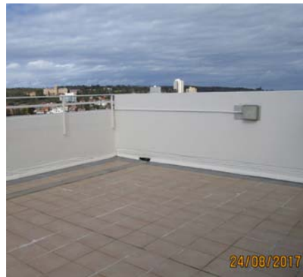
6. Rooftop adjacent to parapet wall
